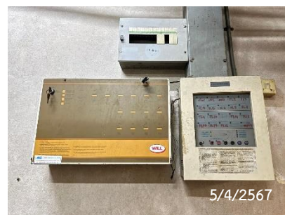
Fire Alarm Control Panel
